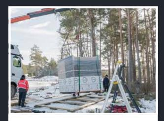
Kirami FinVision® Annex modules are delivered to the installation site as whole units, almost fully assembled.
